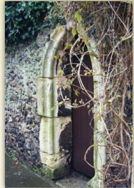
Great Maytham Hall garden wall door
